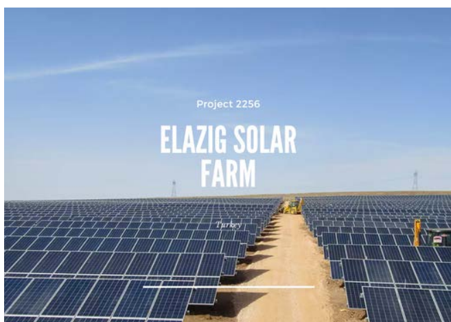
Project 2256: Elazig Solar Farm in Turkey
